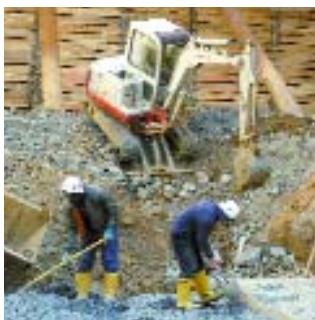
Work is underway at 1717 Rhode Island Avenue, N.W., Washington, D.C.
